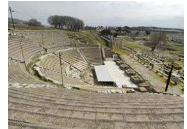
Figure 16: Theatre structure at Asclepieion
