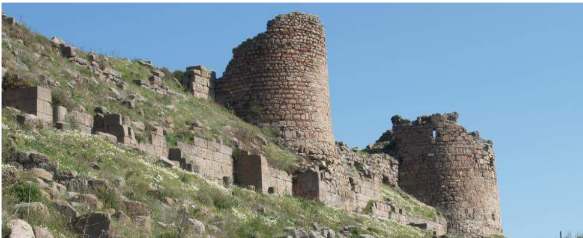
Figure 23: Current situation of the ramparts built in Byzantine Period.
