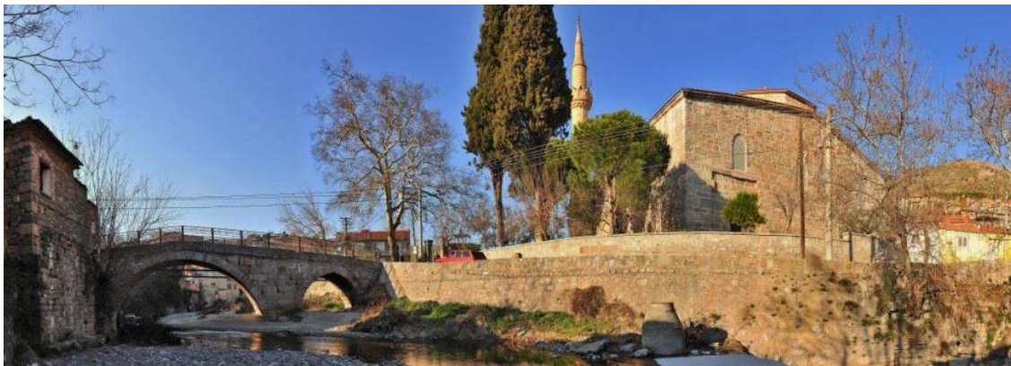
Figure 32: Selinos Brook within Bergama cultural landscape and examples from the bridges over the Brook (Ulu Cami Bridge)
